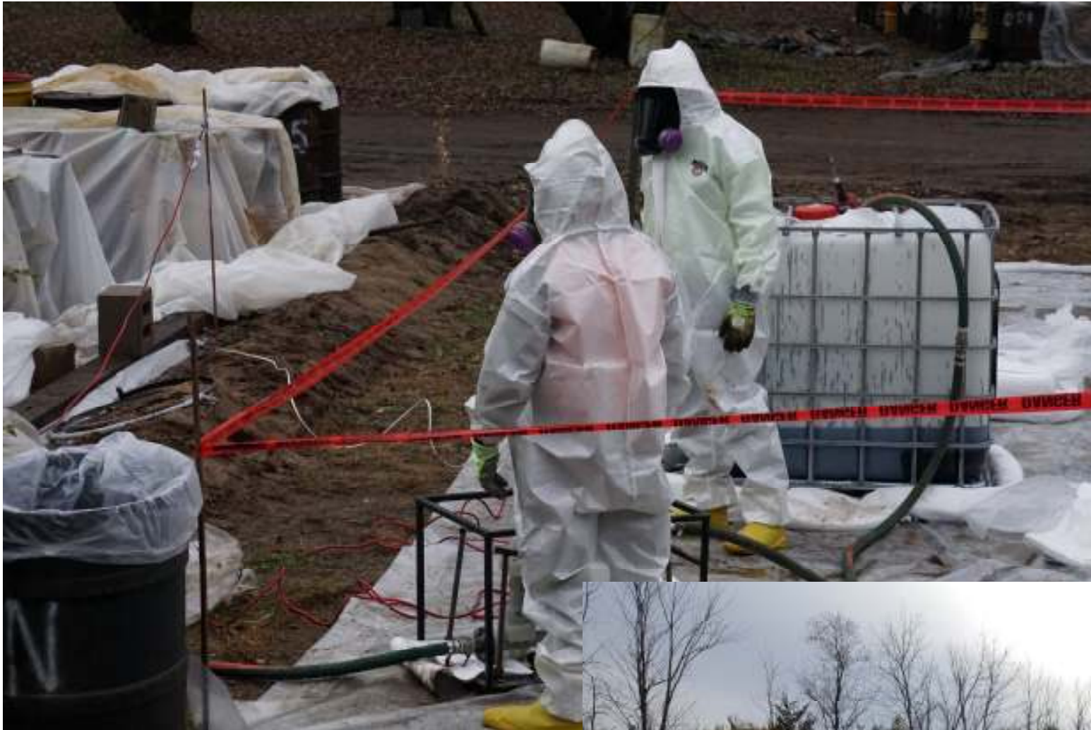
Flammable Liquid transfers and bulking. - Grounding and Bonding
