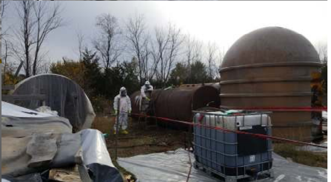
Flammable Liquid transfers and bulking. - Grounding and Bonding
